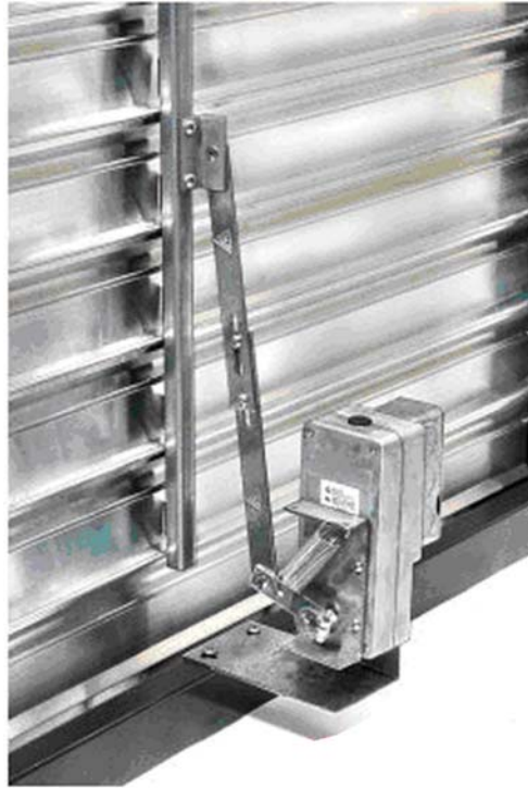
► Shutter Operator close up view.
