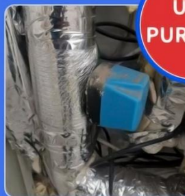
Water tower water supply
