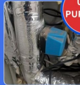
Water tower water supply
